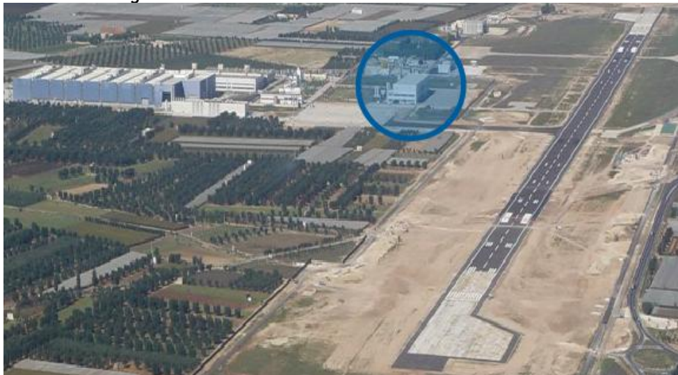
Figure 13. Grottaglie Airport Test Bed (GATB)
